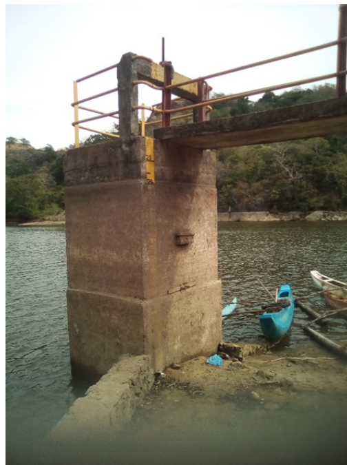
Figure 2: Bissokotuwa of the Buduruwagala reservoir located in the Moneragala District in the Uva Province of Sri Lanka.
